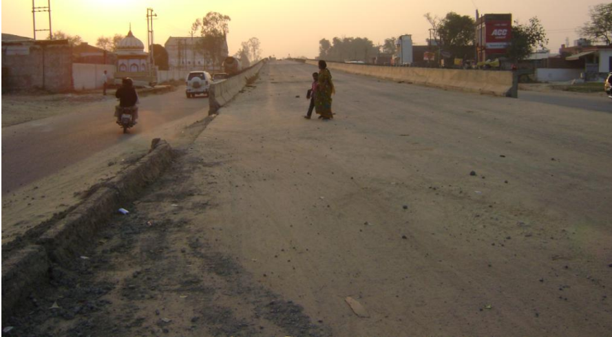
The old dumping site in brick kiln at Ummari village was made empty and Illegally dumped in the slop of Over-bridge at Matiyari Chauraha, Lucknow and road was constructed over it-New picture
